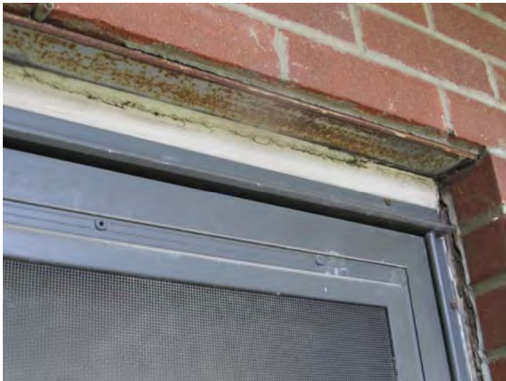
Steel lintels in need of surface prep and painting
