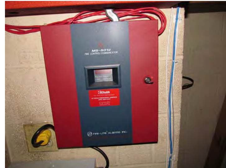
Zone-type fire alarm control panels monitor and supervise hardwired common area end devices
