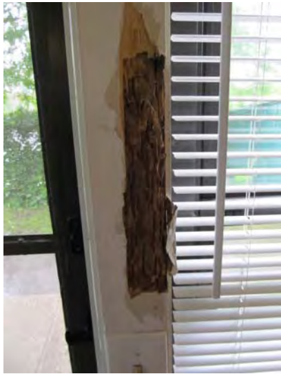
Area of termite damage noted at 'Building 3 – Unit L'
