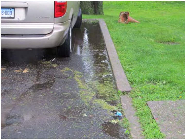
Ponding water noted at some asphalt-paved parking area locations
