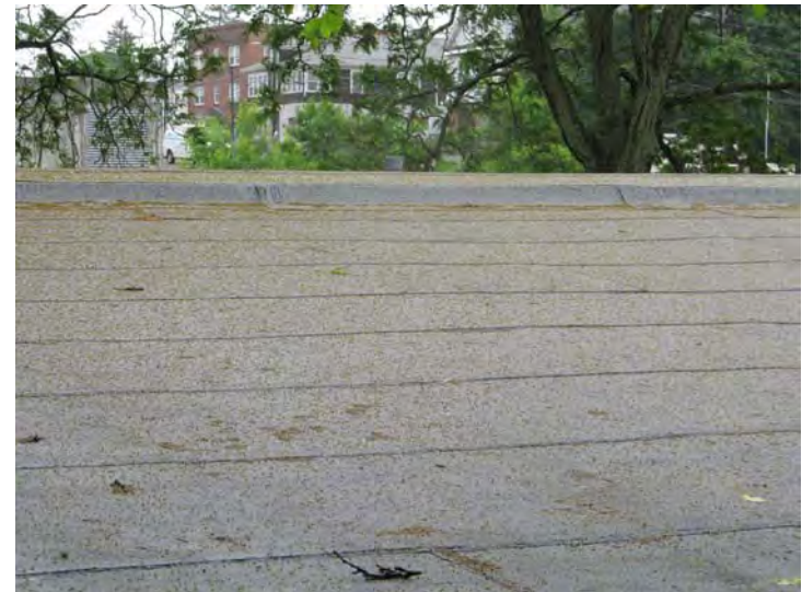
Rolled asphalt roof coverings are in fair condition but approaching the end of their expected useful life
