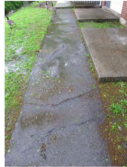
Pedestrian walkways exhibit areas of cracks and ponding water
