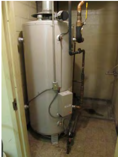
Typical natural gas-fired domestic hot water tank serving a building module
